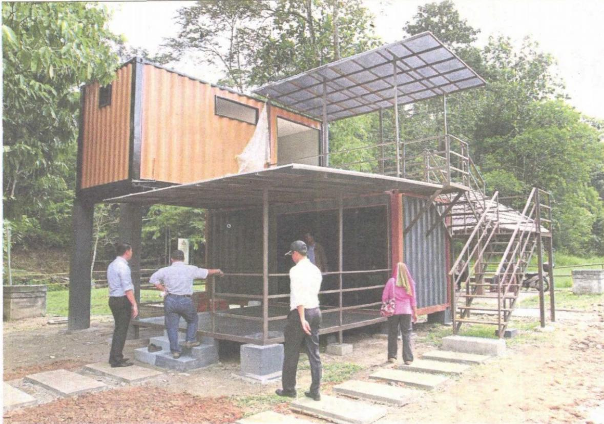
Visitors checking out the double-storey cabin, which can accommodate four to six people, is made from used shipping containers.
